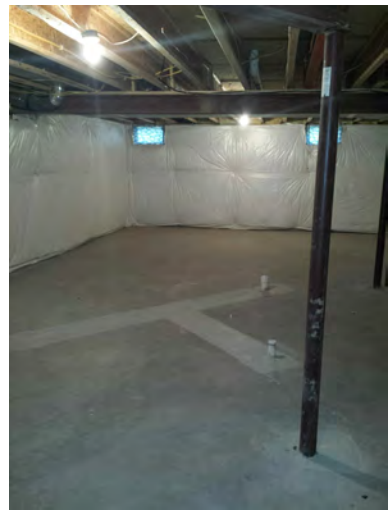
HVAC and Hot Water
