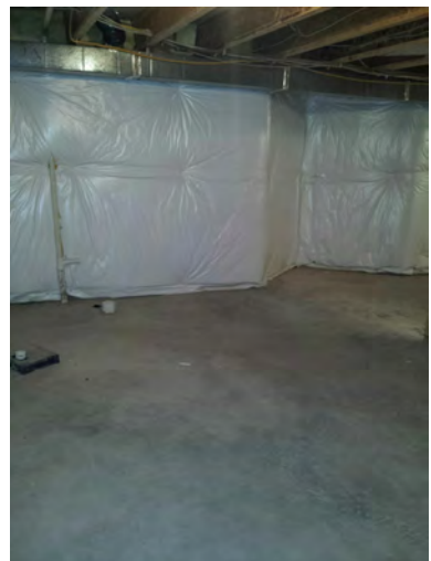
HVAC and Hot Water
